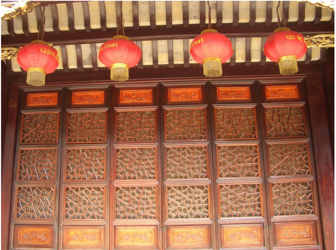
Fig. 4 Chinese lattice constructed from multiple identical blocks
